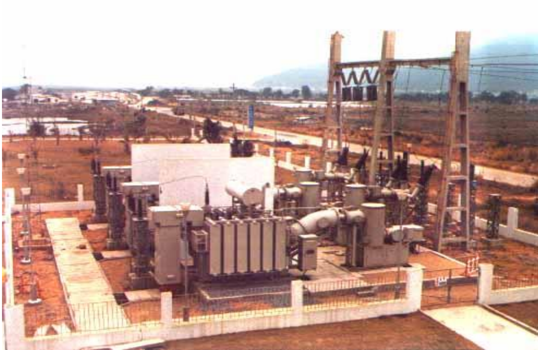
The 110KV Power Station with 3 main-transformers 121 KV/11KV, 47 MVA and the 110 KV GIS
