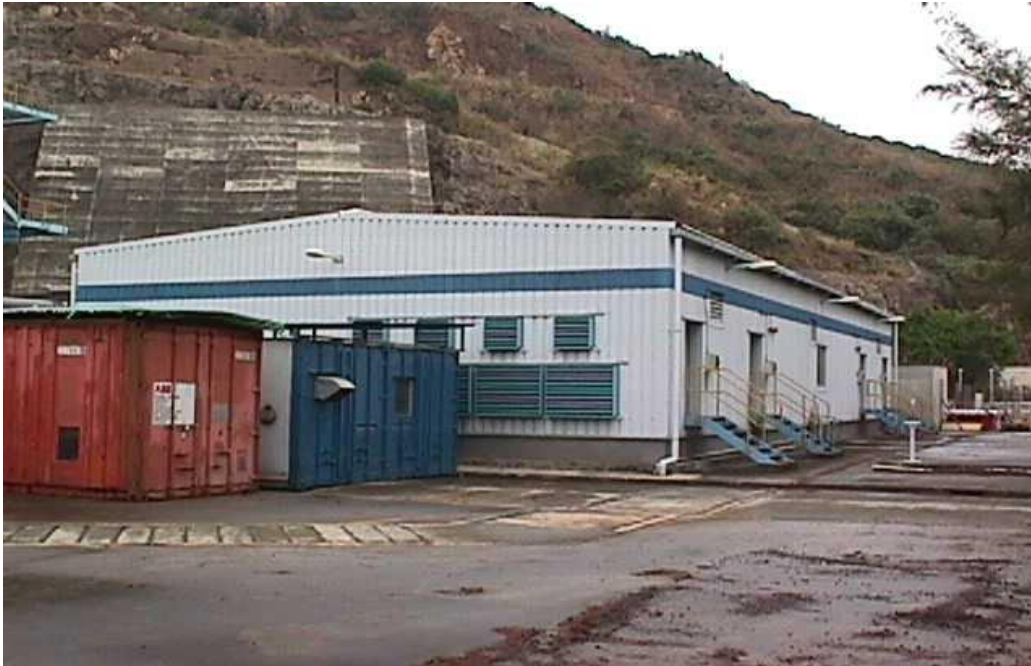
Control Room Package
