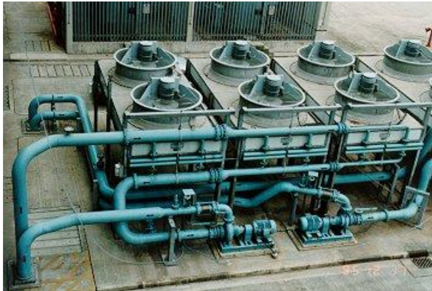
Generator cooling water skid
